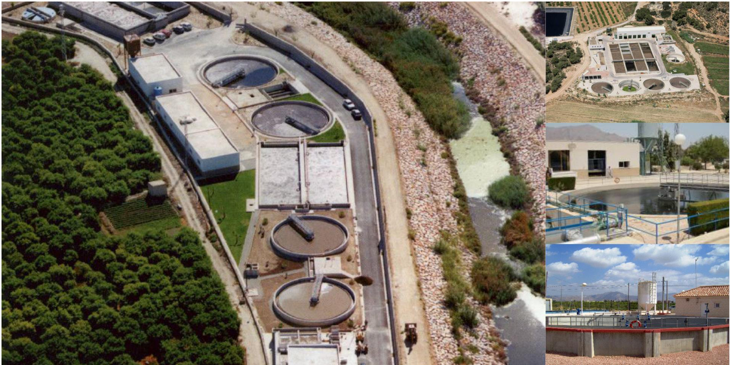
reinforced concrete structures for sludge digesters and primary
